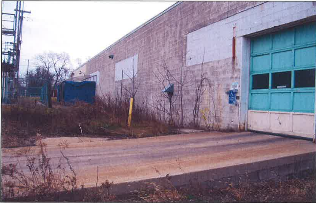
PHOTO NO. 3: View of north side of building.
