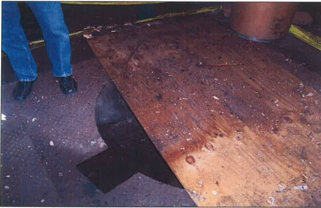
PHOTO NO. 13: Former draw furnace area, with in ground pit.
