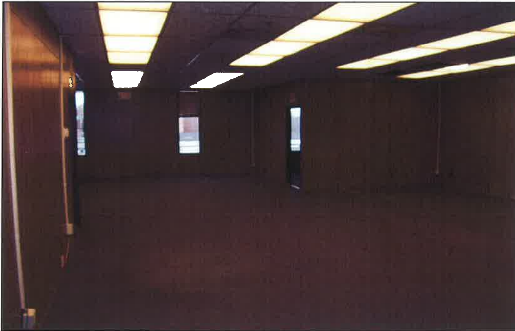
PHOTO NO. 10: Interior second floor office space.
