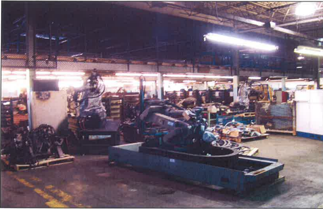
PHOTO NO. 23: Mezzanine area and former vapor polisher area.
