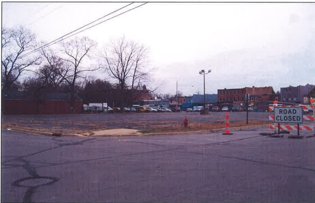
PHOTO NO. 4: View of east parking lot parcels on Property and east adjoining properties (in background).
