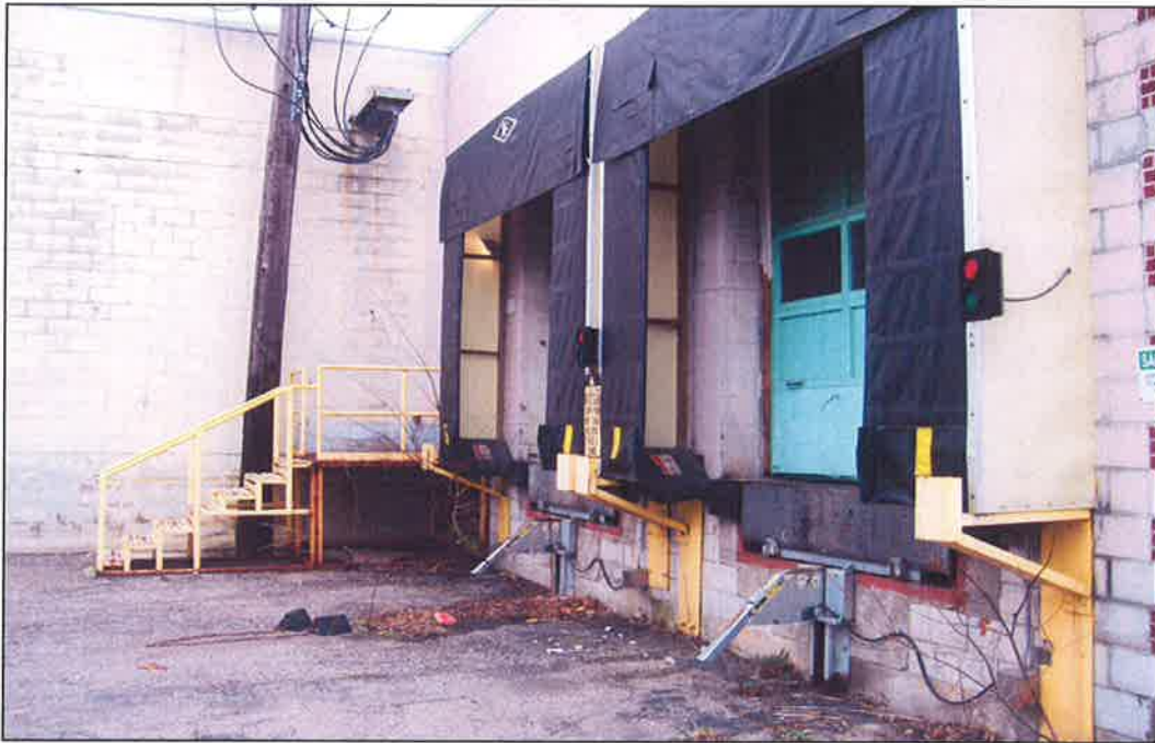
PHOTO NO. 18: Southern loading dock area.
