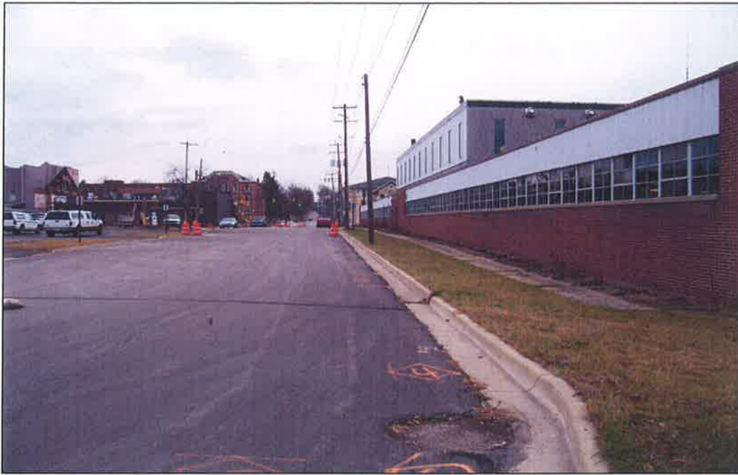
PHOTO NO. 1: View of east side of building.
