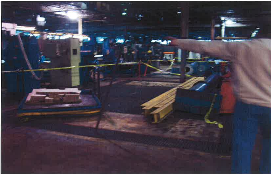
PHOTO NO. 12: Coolant catch pits.
