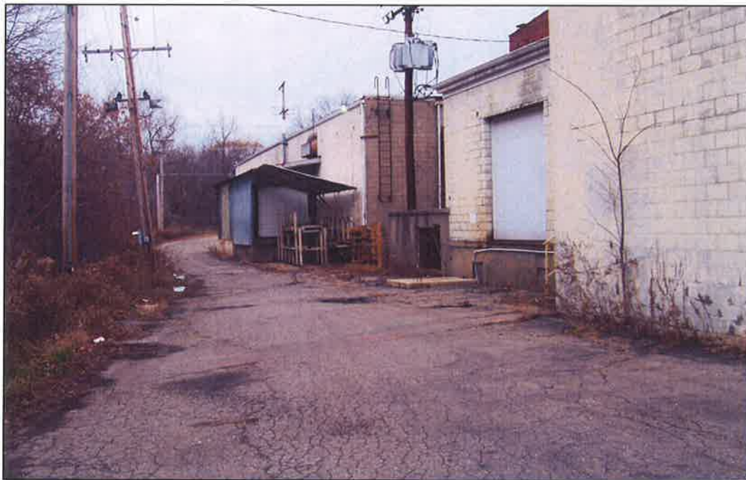
PHOTO NO. 20: Reported trichloroethylene dumping area (adjacent to loading dock).
