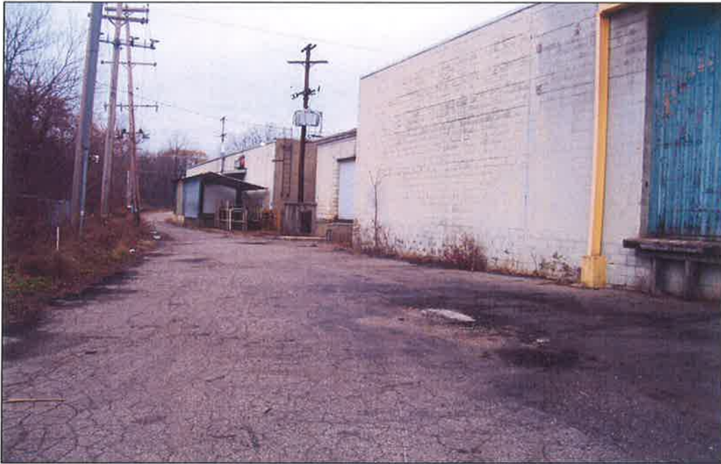
PHOTO NO. 9: Pole-mounted transformers on west side of Property.
